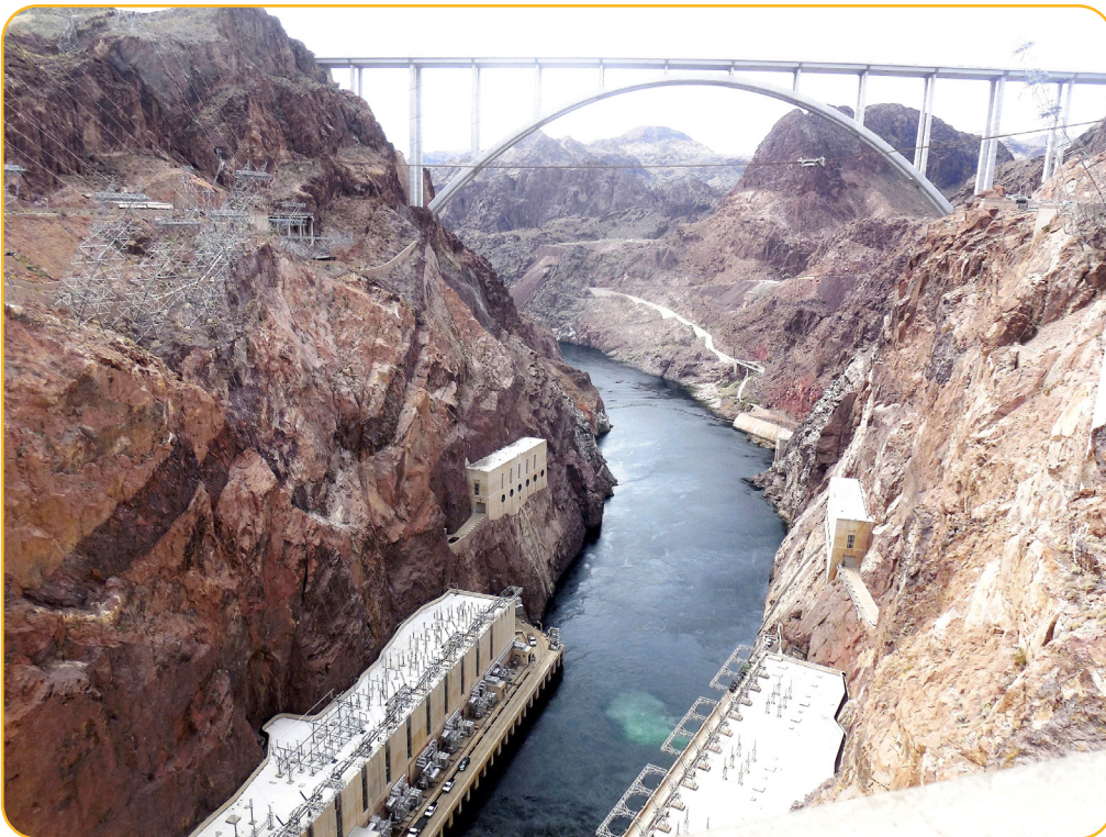
Hoover Dam in the black canyon of the Colorado River on the border of Arizona and Nevada (US).
