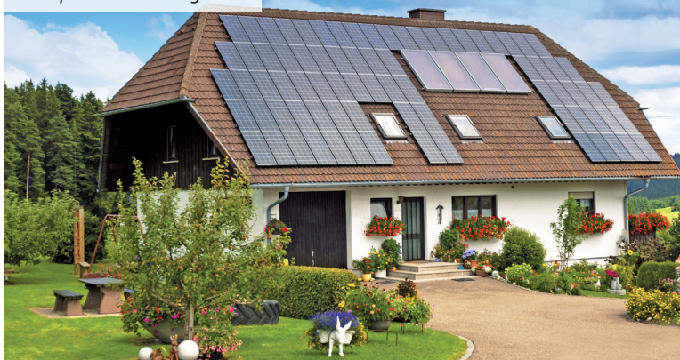
Solar panel on a cottage roof
