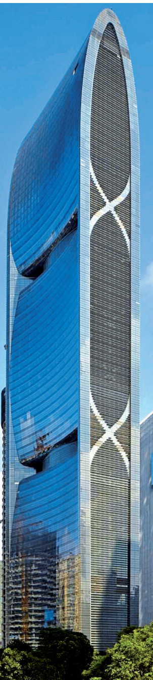
Pearl River Tower, Guangzhou (China) is one of the world's most energy-efficient skyscrapers. It uses wind energy and solar technology.
