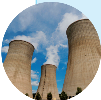
Nuclear cooling towers
